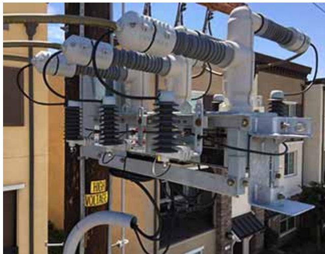
Figure AP 510-10: Surge Arresters for Recloser Installations
