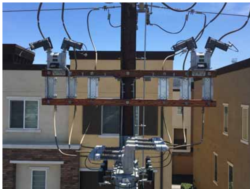
Figure AP 510–6: CPT Riser Details for Option 1
