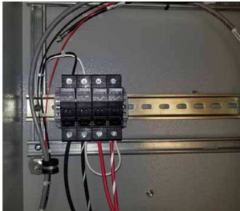
Figure AP 510–11: 120 V Control Power Connections
