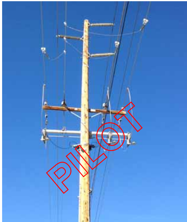
Figure 620P-18: Typical Installed Configuration of Lineprobes Using Hotline Clamps for Neutral
