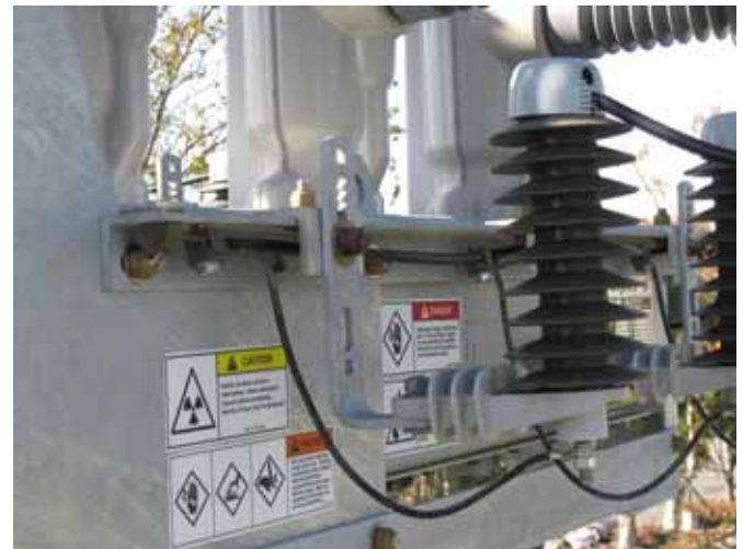
Figure AP 510-10: Surge Arresters for Recloser Installations
