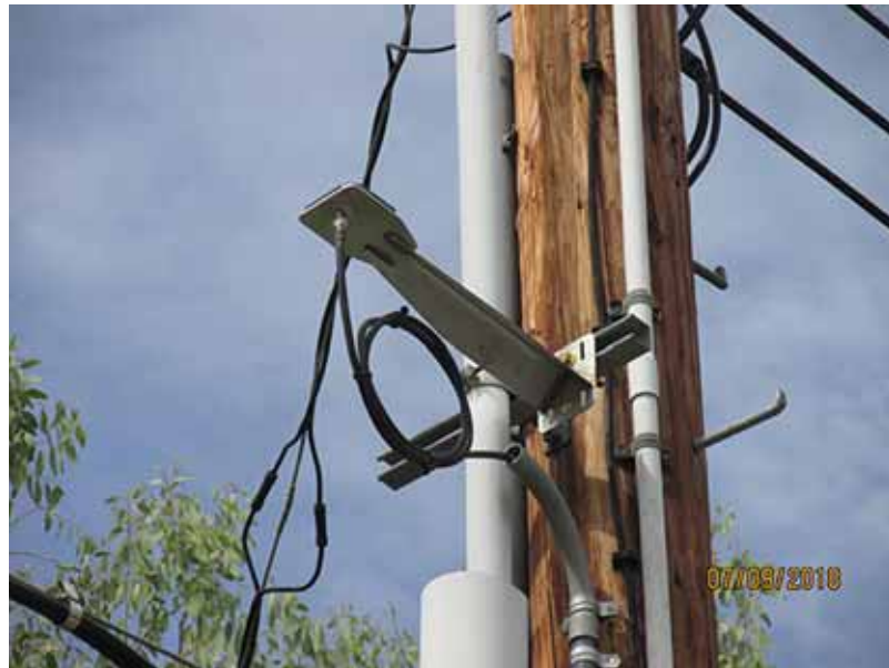
Figure 620P-9: Complete Installation of Antenna Extension
