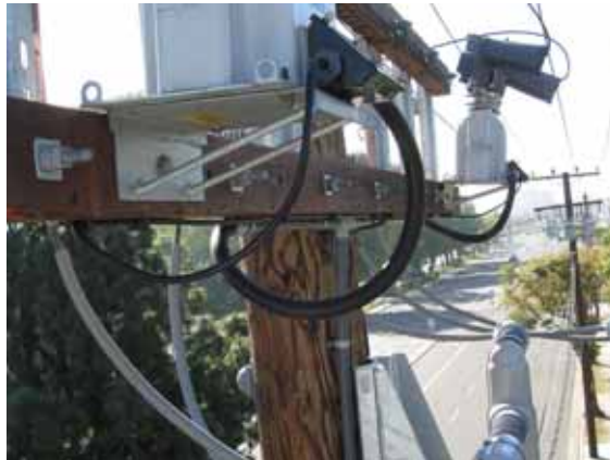
Figure AP 510–7: CPT Riser Details for Option 2
