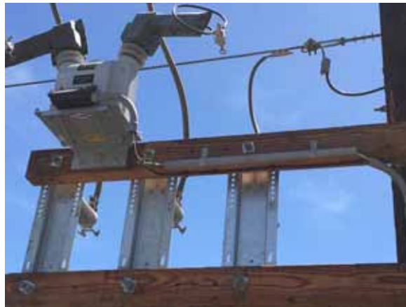
Figure AP 510–8: CPT Grounding Details for Option 1
