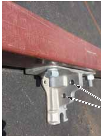
Figure PO 370–2: Composite Crossarm Mounting Bracket with Guy Attachment Holes
