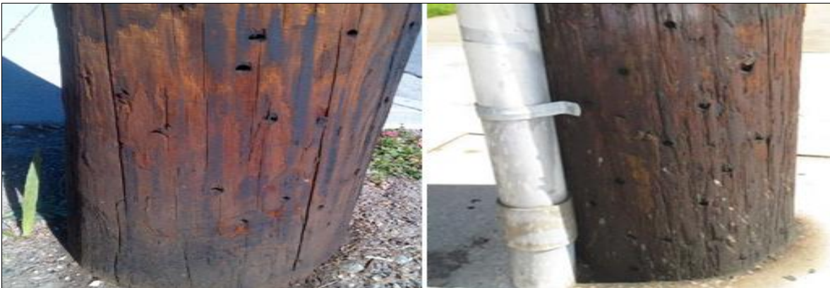
Photo 4.1 and 4.2: Through-bored Poles
