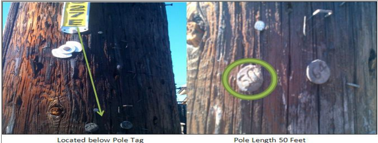
Photo: 4.13 and 4.14: Location of Nails and Length nail
